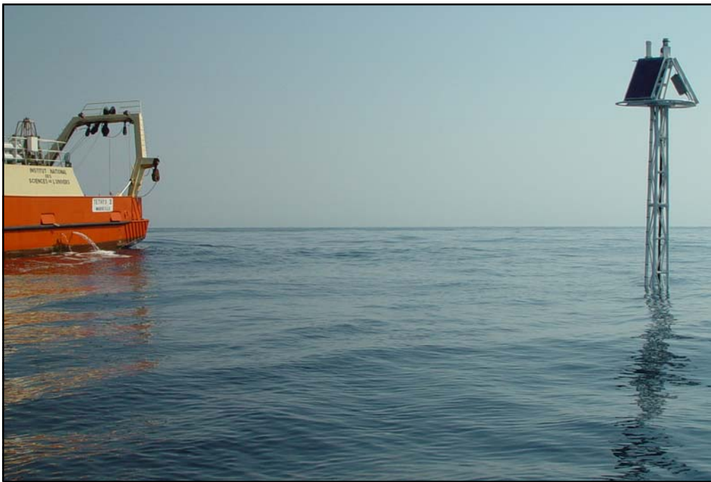
Fig. 10b. The buoy completely deployed with the top-most portion of the structure rising approximately 4 m above the water surface (as measured from the bottom of the solar panels).
