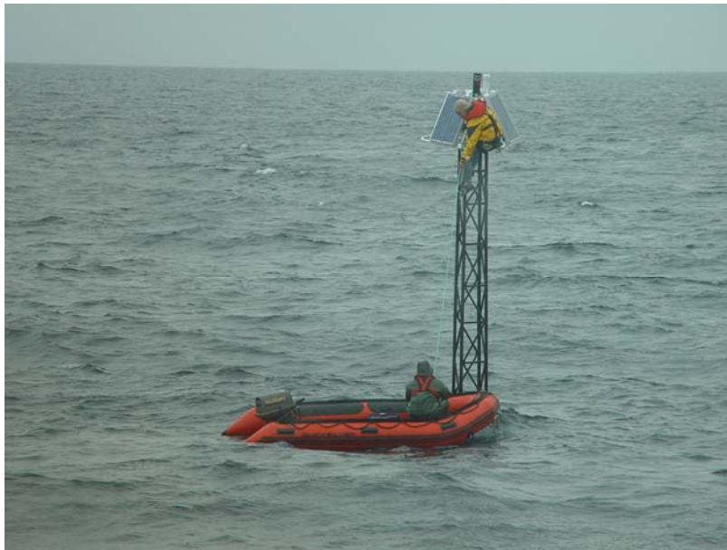
Fig 1. Hoisting materials up to the Boussole buoy head to attempt a direct communication link with a laptop PC.
