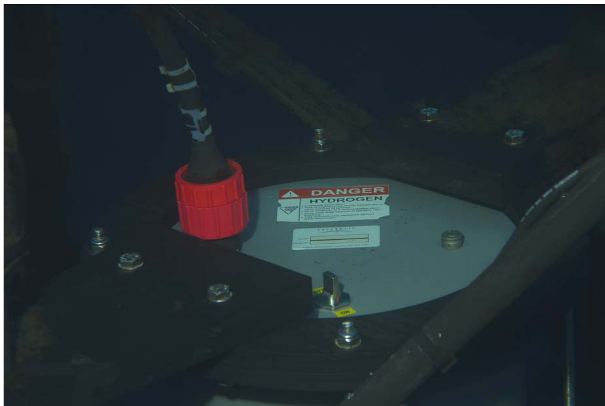
Figure 1. The buoy battery was taken off the buoy, recharged during one day and put back on the buoy by divers.
